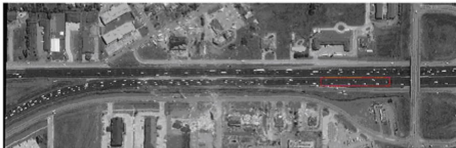
Figure 3.2.4: Highway in Oklahoma
