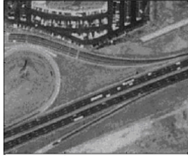
Figure 4.4.1: Highway in France
