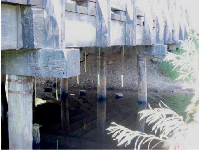
In general, measured vibrational frequencies of single-span bridges have been observed to range from 17.5 Hz to 35.0 Hz. Bridge stiffnesses ( $EI$  as measured with static-load) ranged from 5,100 to 200,000 ( $10^6$  lb-in<sup>2</sup>), and show a quadratic increase with measured fundamental frequency, as the models of this study substantiate [40].
