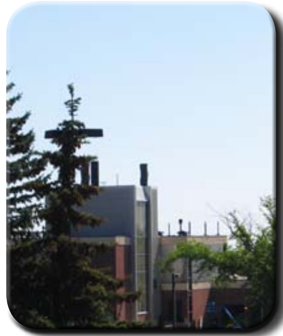
Lund Heating Plant keeps the campus comfortable during the summer and frigid winter
