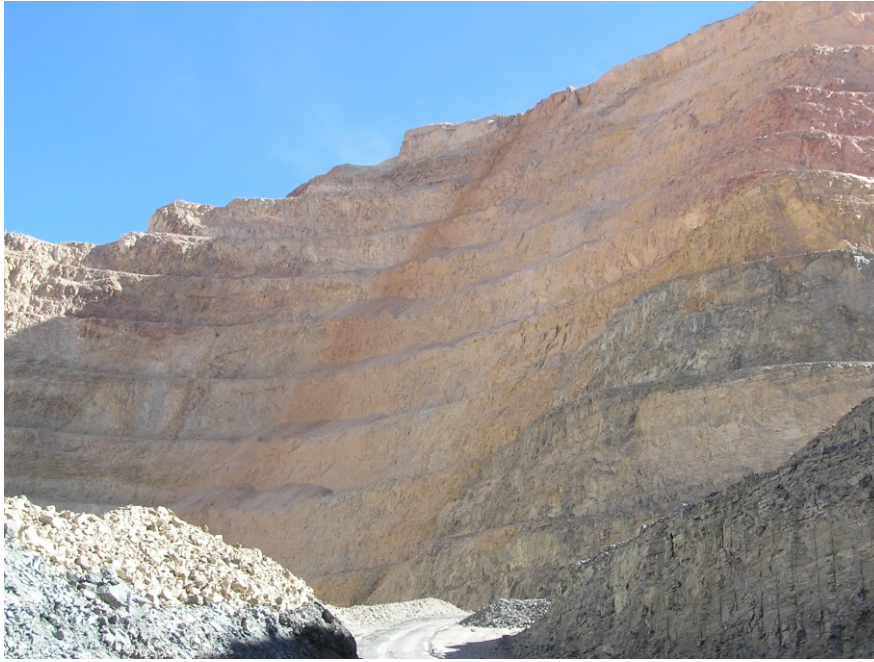
Figure 9. View of a benched slope in an open pit mine used to illustrate the application of the computational tools for stability analysis presented in this paper.
