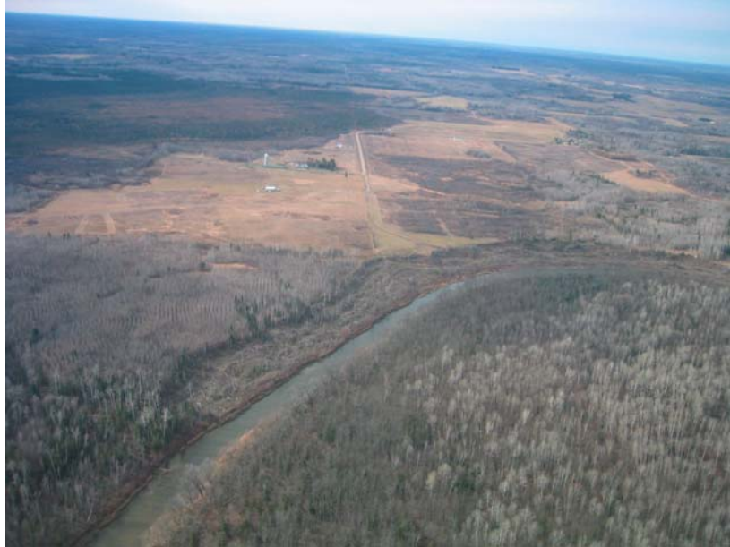
Figure 0.2: Large rotational failures and slumps extending up to the top of the slope break on the outside of a bend.
