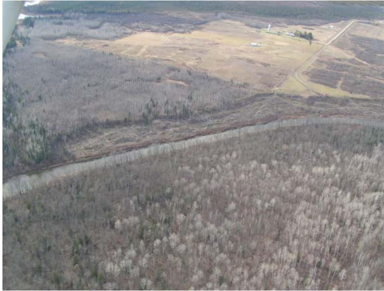
Figure 2.14: The outer edge of a meander bend has slumps reaching up to the top of the slope break.
