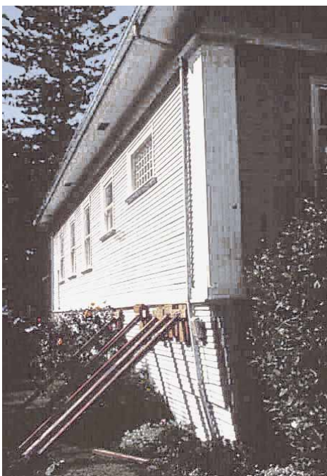
This home in Santa Cruz, California, damaged in the 1989 Loma Prieta earthquake, shows the effects of a weak "cripple-wall" connection between the upper part of the house and its foundation. Houses without adequate connections to foundations can easily shift during even moderate earthquake shaking, causing extensive damage. For example, pipes and wires may be broken by a slight cripple-wall shift, resulting in fires, water damage, or other problems. Much damage of this type can be avoided by using inexpensive bracing techniques, such as those recommended in the seismic design provisions of building codes.
