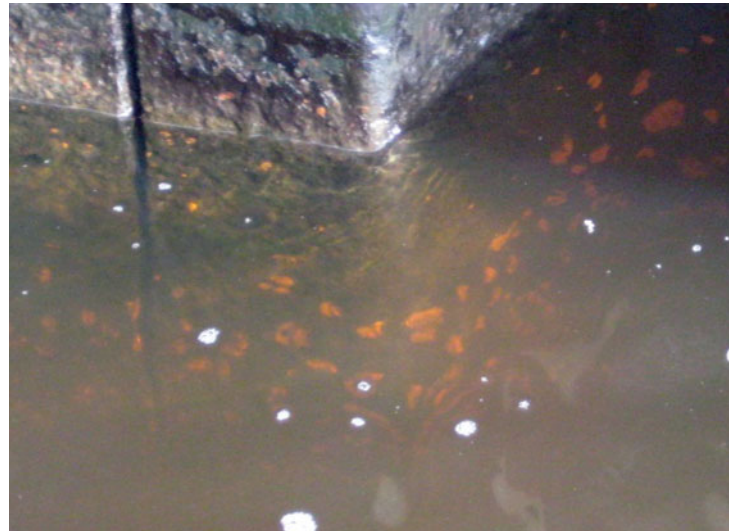
Corrosion pitting and tubercle formation at Hallett Dock 5.
