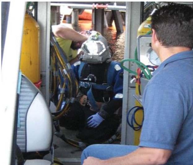
AMI consulting engineers Chad Scott and hard hat diving team at Midwest Energy Resources.
