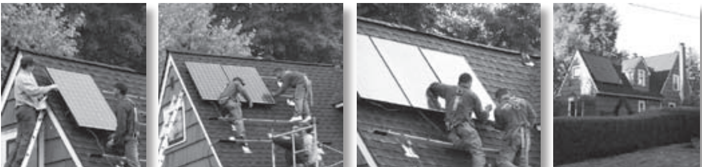
Shown above is a GTS 597 package utilizing Sanyo 190 watt modules that was completely installed by a crew of three in less than a day.
