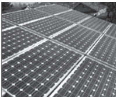
Modules interconnected together are called a sub-array and these connected together comprise a total solar array
