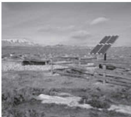
Grundfos SQ Flex water pumping system in Southern Wyoming
