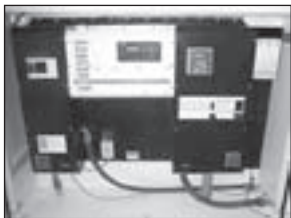
SunWize Power Center
