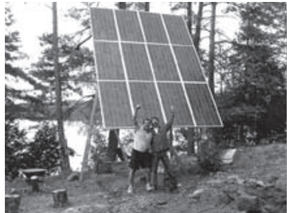
1980 watt system using 12-Sharp 165W modules powers a remote home in Canada. Installed by Quality Solar.
