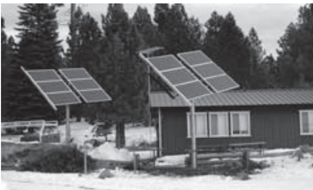
1980 watt system utilizing 12-Shell SQ165W modules and an SMA 1800 inverter. System installed at Lassen Volcanic National Park in Northern CA.
