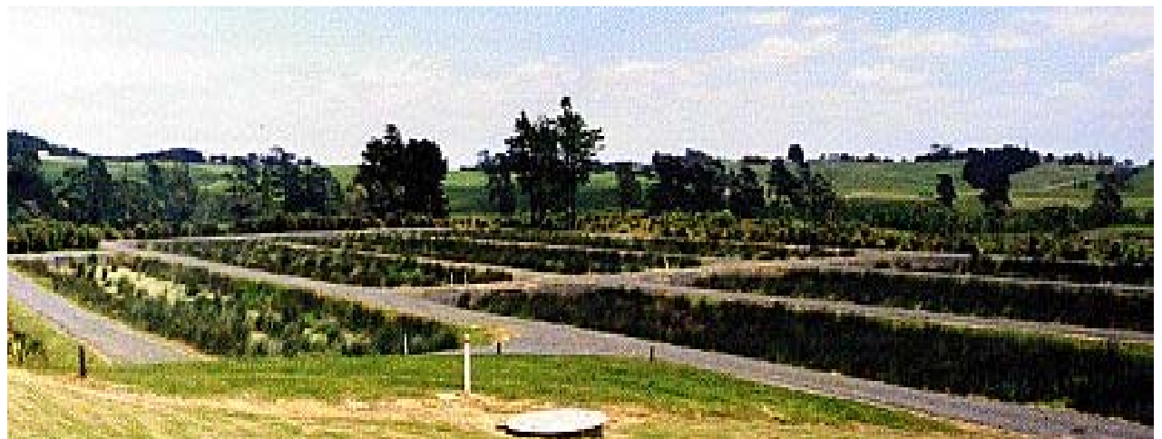
Photo 4: Surface-flow wetlands providing tertiary treatment after aerated lagoons at Beachlands-Maraetai. The final discharge is UV disinfected and dispersed into restored wetland and pond areas that drain to a nearby stream.
