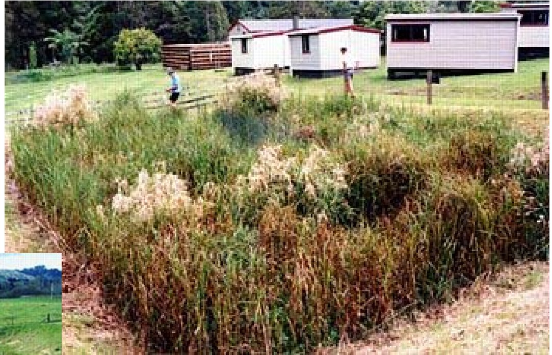
Photo 2: One of two small subsurface-flow constructed wetlands receiving motor camp wastewaters after septic tank treatment at Waipoua Forest Park.
