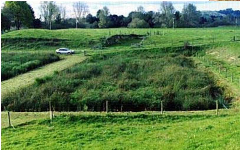
Photo 3: One of three gravel-bed subsurface-flow wetlands treating sewage from Waikeria Prison after the activated sludge treatment
