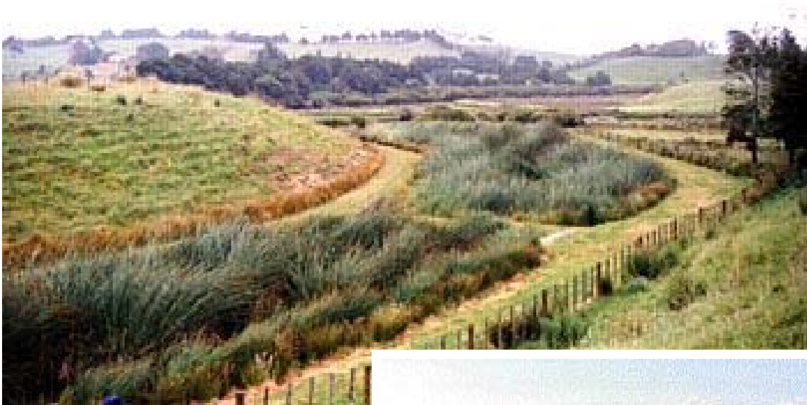
Photo 1: Surface-flow wetlands providing advanced secondary treatment at Kaiwaka after 2-stage waste stabilisation ponds.
