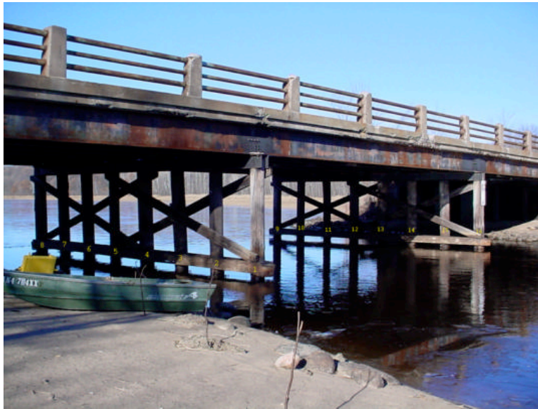
Figure 5. Mn/DOT District 1 bridge 5919 showing the 16 timber piles that were tested.
