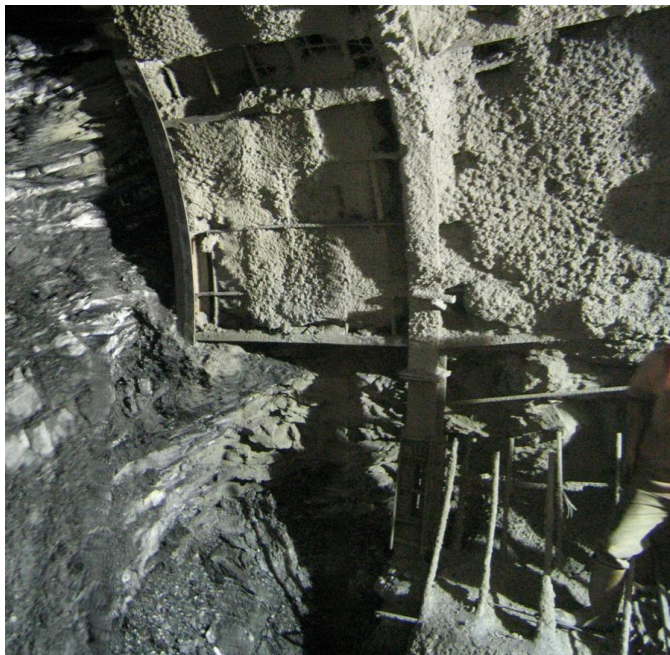
Figure 32. a) Configuration of mid-height bench (partially disintegrated in this photograph) and upper steel arch installed ahead of lower section and sliding joint. b) Final 60 cm section with outer shotcrete and steel set composite section and inner reinforced shotcrete section. The tunnel is to the left and rock mass is to the right of the section.
