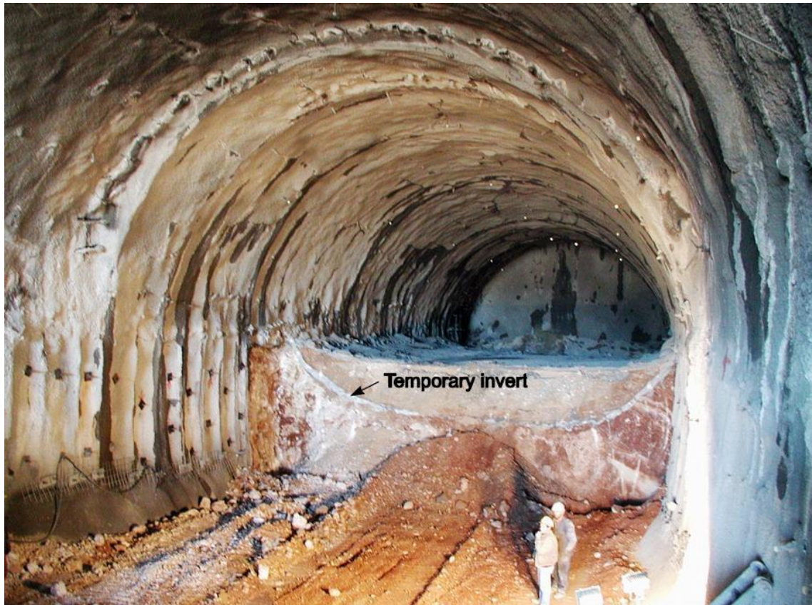
Figure 15. Top heading and bench excavation in a weak rock tunnel where a temporary shotcrete invert was used to control floor heave.
