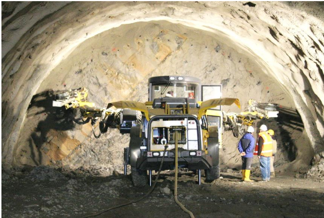
Figure 9. A simple top heading shape in good quality interbedded sandstones and siltstones. The tunnel arch is supported by means of rockbolts and a layer of shotcrete and no face support is required. The flat floor requires no special treatment other than good drainage of surface water accumulations.
