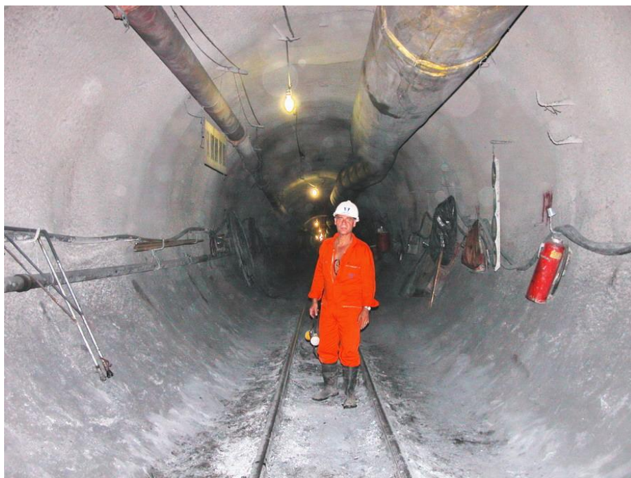
Figure 39. Completed section of tunnel with a 60 cm thick reinforced shotcrete lining, placed in two layers as described above.
