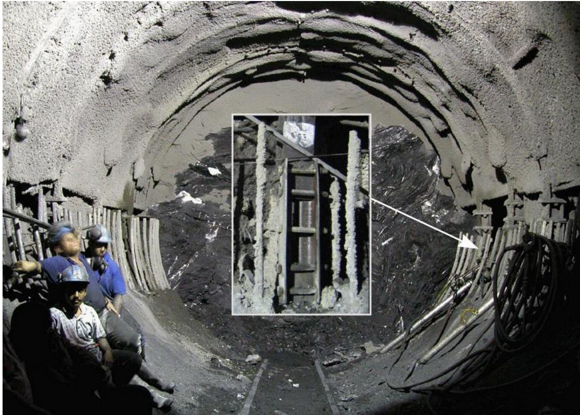
Figure 31. Initial Liner composed of circular steel arch and 20 cm of shotcrete. Inset shows detail of sliding joint with shotcrete gap. Note rebar in place to reinforce final shotcrete layer.
