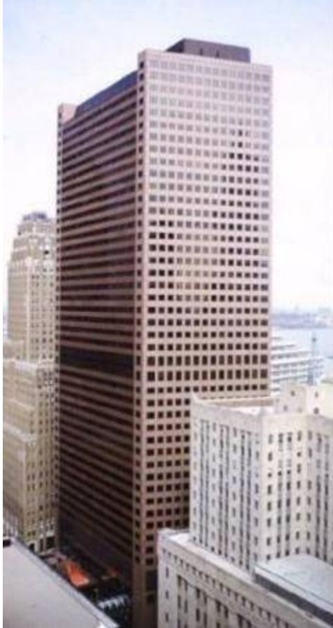
WTC 7: 47 - Story, steel-frame building..
