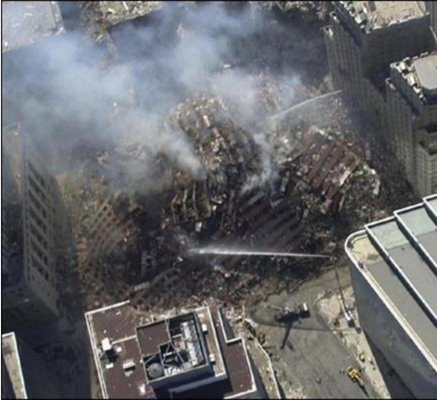
WTC 7 collapsed completely, onto its own footprint
