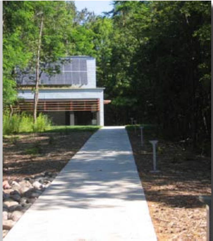
Solar lighting along the pathway
