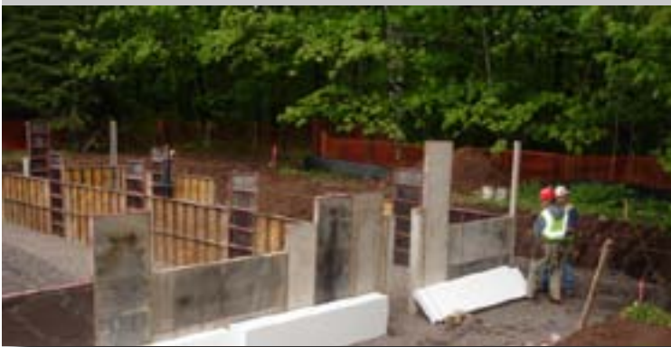
View of the foundation, early in construction
