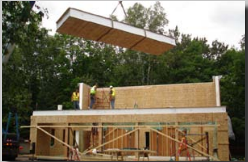
Installing SIP panels, August 2009
