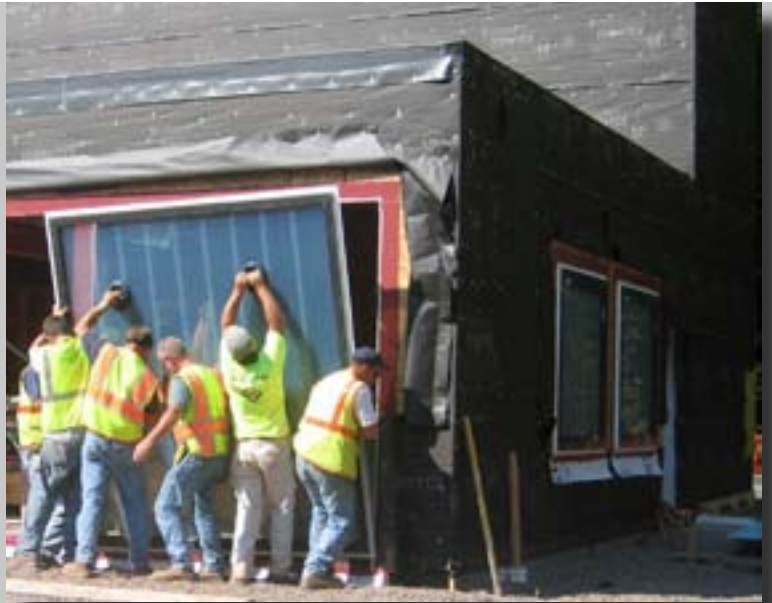
Installing triple pane windows, September 2009
